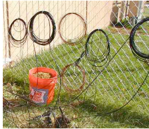
Figure 7. Coiled sensor cables stored off the ground.
