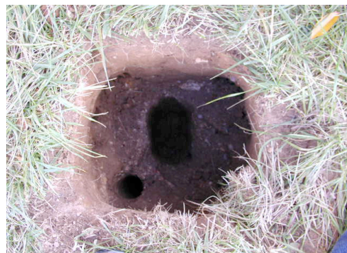
Figure 4. Excavated installation pit.
